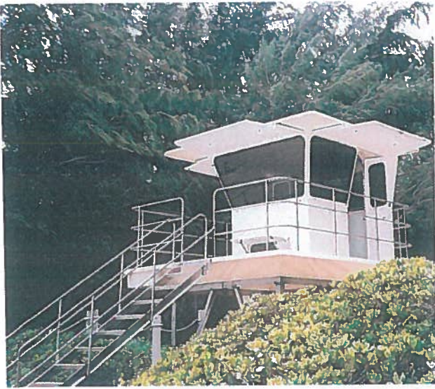
Waimea Bay Beach Park, Oahu, Hawaii Permanent site stainless steel structure, 35 degree low angle stairs.
